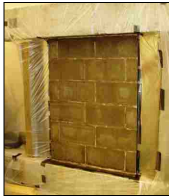
(a) Primed URM Wall
