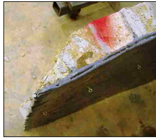
(b) Damage Sustained to WF-FA Units
