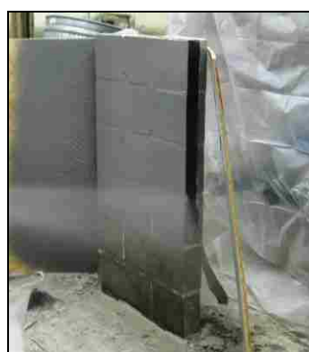
(a) Initial Polyurea Layer
