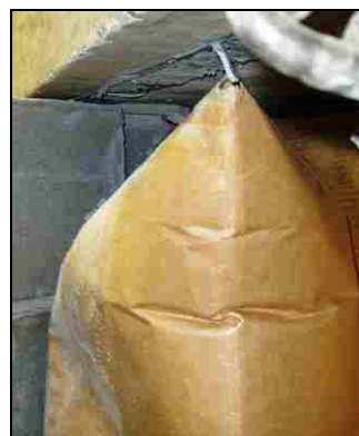
(b) Debonding of Polyurea
