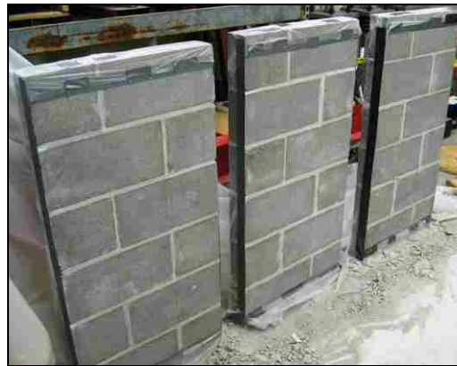
Figure 6.2. Phase 2 URM Walls Prior to Strengthening
